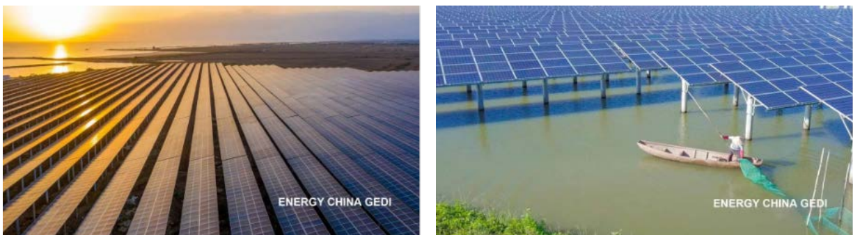
Figure D4. 500 MW Fisheries Photovoltaic Power Generation Project in Haiyan, Taishan
